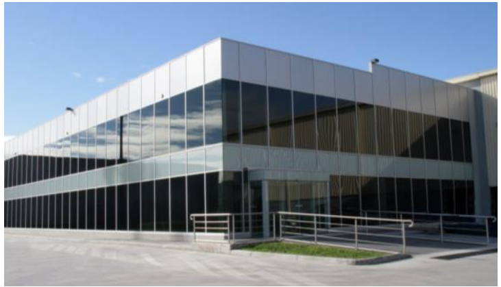
Glassworks Pty Ltd. Dandenong Victoria, Australia
