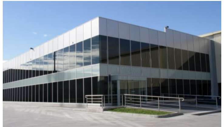
Glassworks Pty Ltd. Dandenong Victoria, Australia
